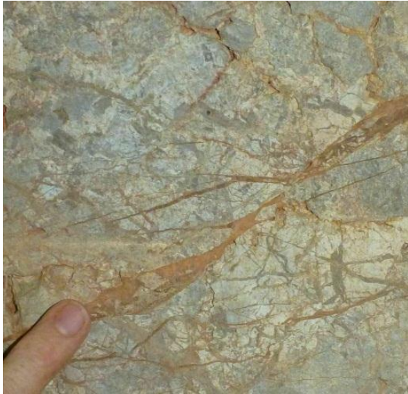
Micro fractures in the solid walls
